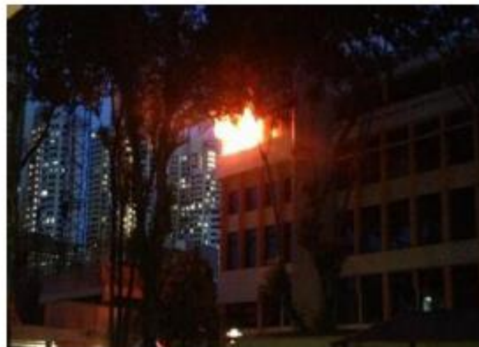
Office Fire at Singapore Polytechnic, Teaching Block 2, Level 5, July 16, 2013 ~7:25pm
