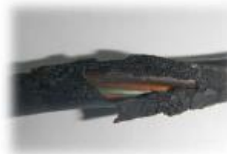
Damaged insulation of an electrical cord
