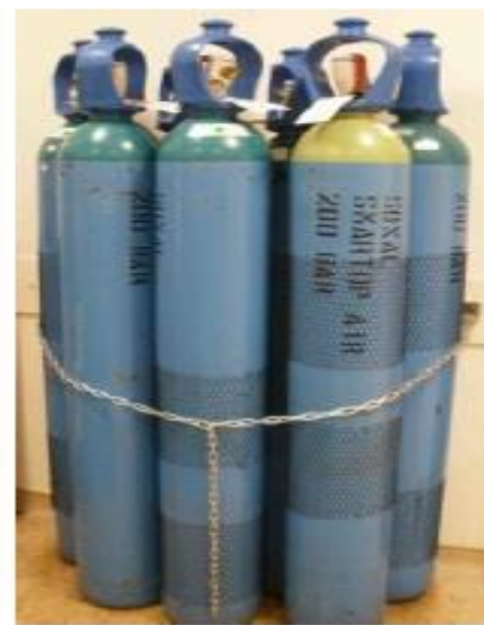
wall bracket – incorrect (one chain – many
